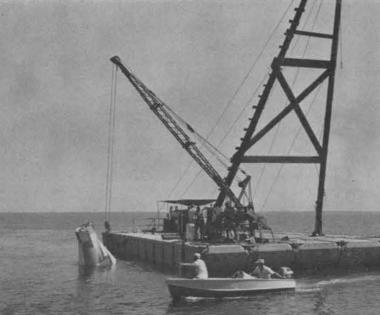
FISHING the Project Mercury capsule out of the water is the Sandia barge and launch at Salton Sea Test Base. A test has just been completed and the recovery of the one-ton capsule is under way. Men of 4580 perform this operation. Thirty-seven drop tests of the capsule have been completed. Photo by Harley Moody (5262).
